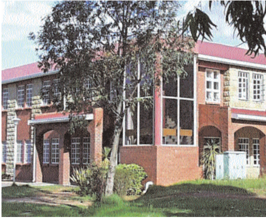
Recently completed Faculty of Science Block
